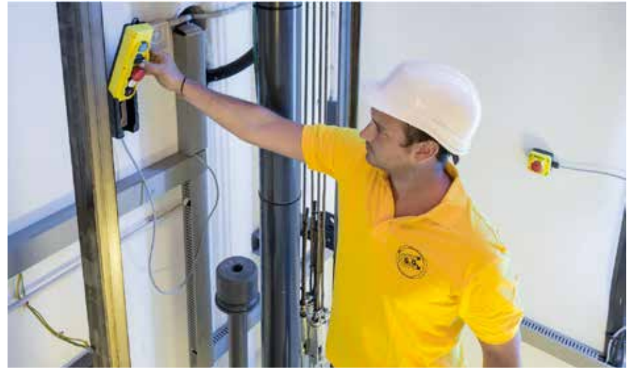
Pit inspection Station
